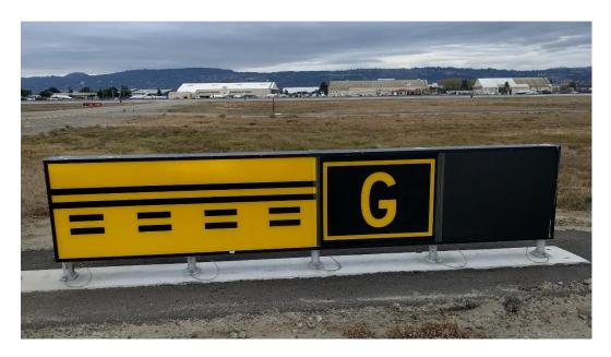
The Airfield Signage Replacement Project will install new and provide upgrades to over 200 airfield signs including installing new airfield sign foundations with new base cans; new and replacement signage; new conduit and conductors and other electrical infrastructure as well as bird deterrent spikes onto all new airfield signs and existing airfield signs.
