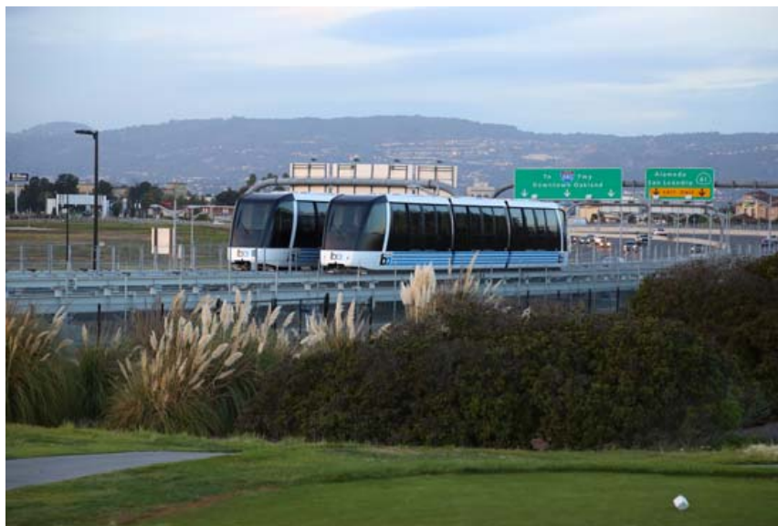
BART Oakland Airport Connector. Source: BART.
