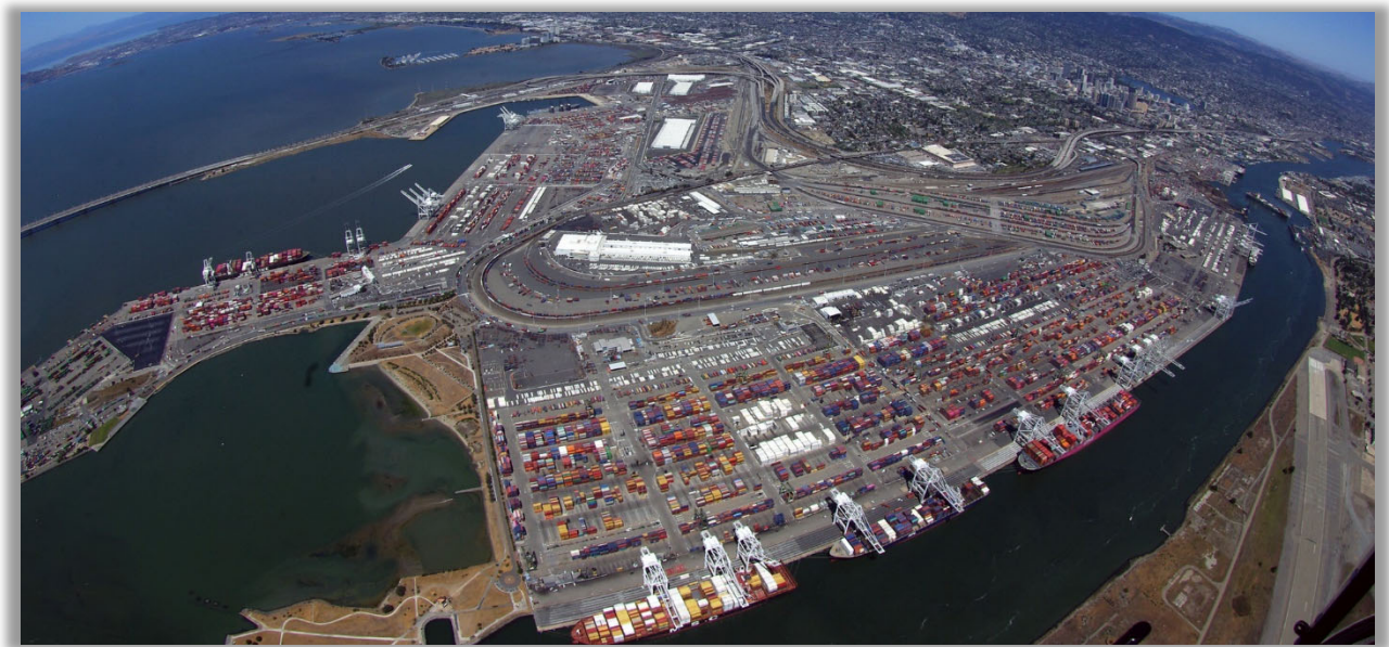
Aerial view of Seaport Facilities at the Port of Oakland
