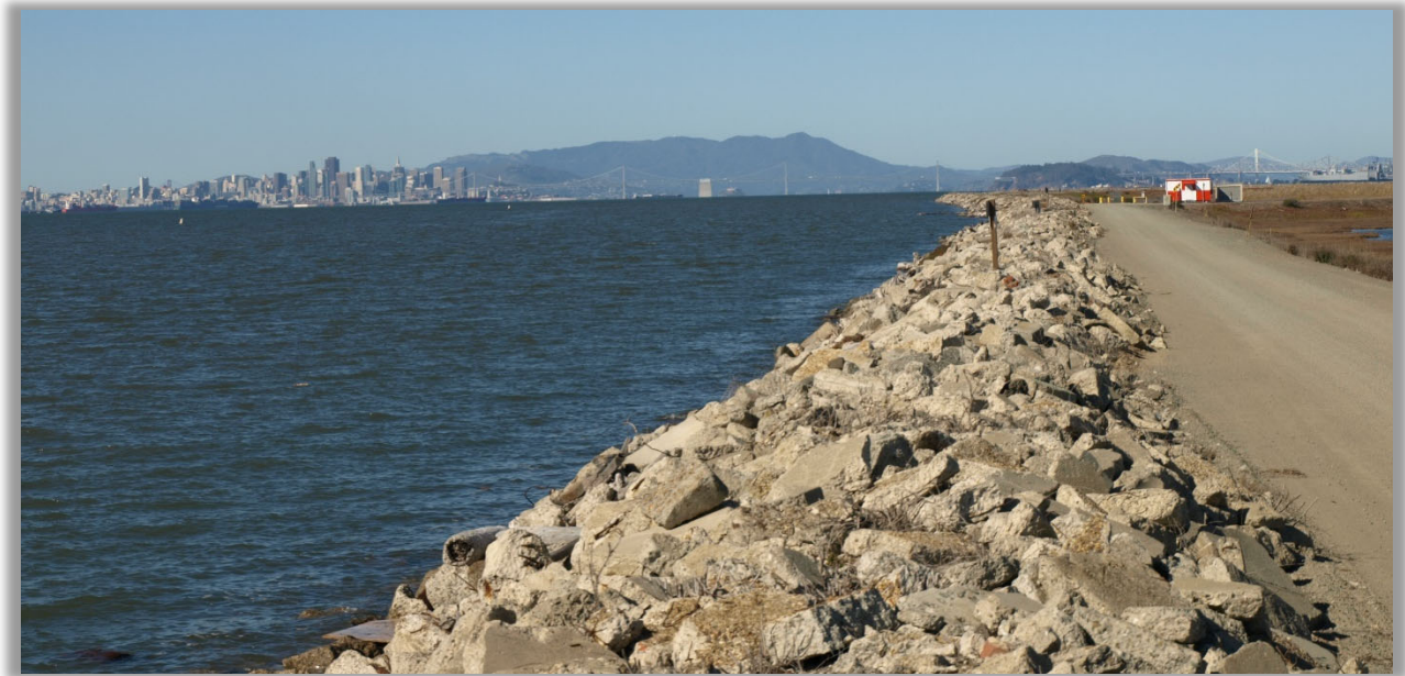
OAK Airport Perimeter Dike
