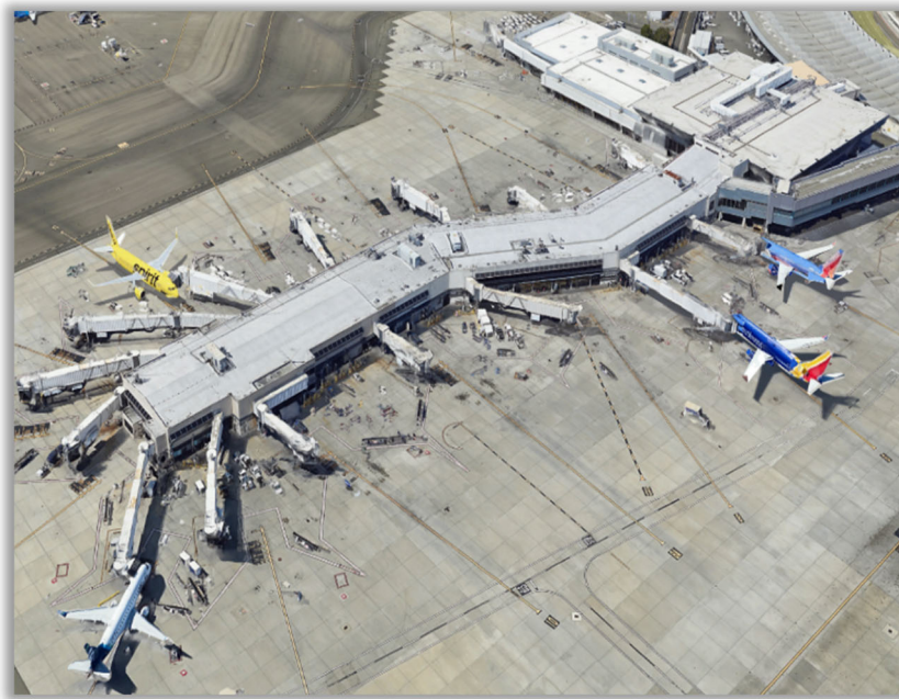
Aerial View of M103 Roof
