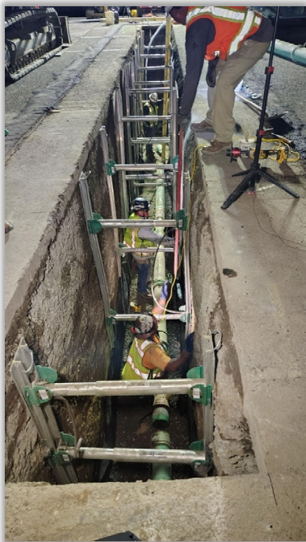
Sewer undergoing repairs at OAK
