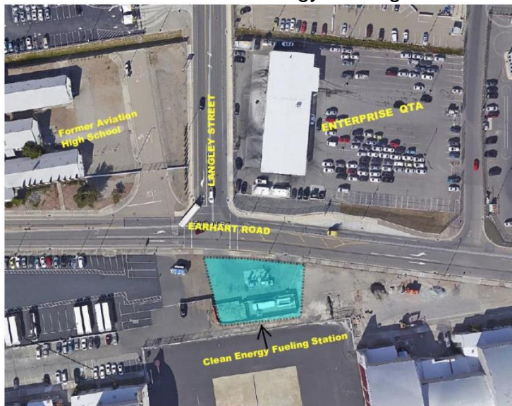
Location of Clean Energy Fueling Station
