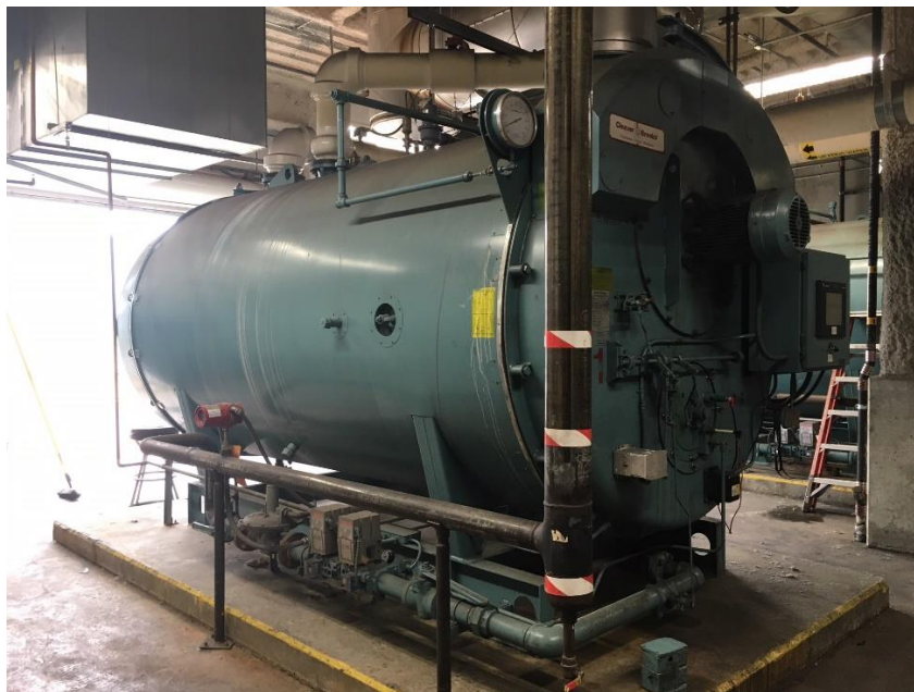
Figure 1 – Existing Terminal 2 natural gas fired boiler.
