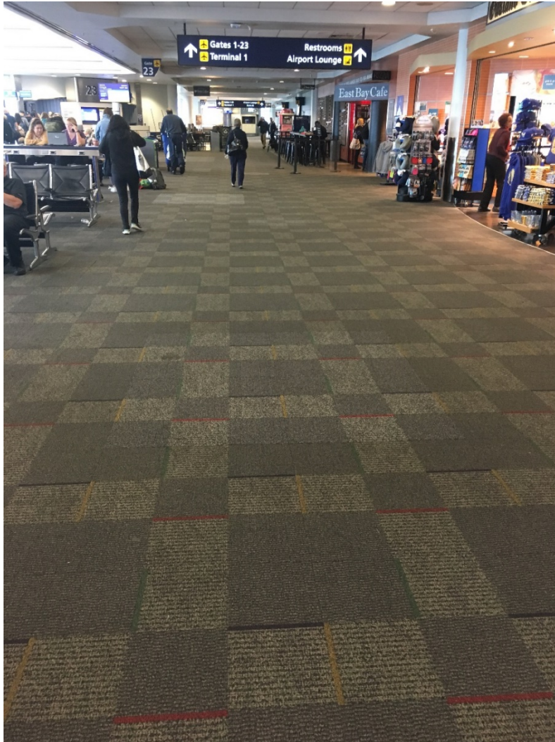
Figure 2. Existing carpet flooring in OAK Terminal 2 concourse (M-130).
