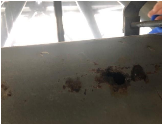
Photo 2: Deteriorated Drain Pipe
